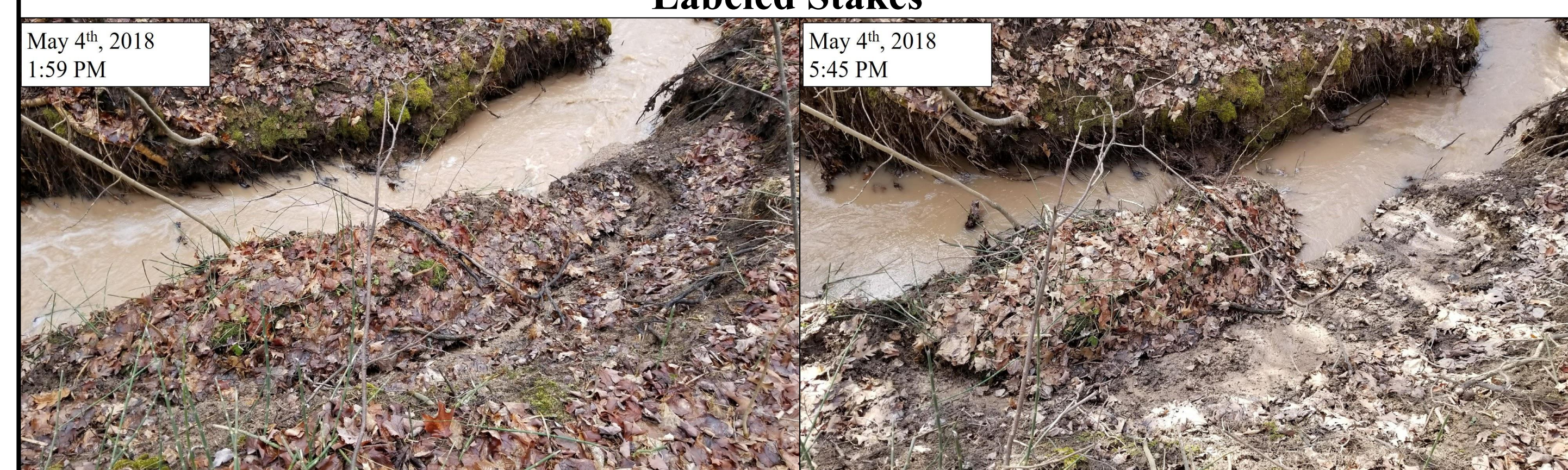
*Figure 11 - Observational Slumping (Near Location #2)
